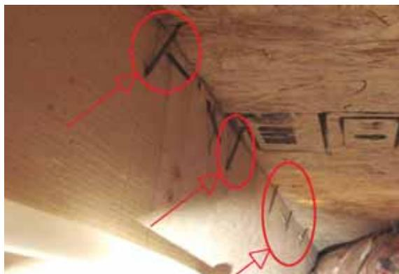
Fasteners missing joists create squeaky floors and expensive callbacks. AdvanTech flooring’s patented fastening guide helps you do it right the first time.
