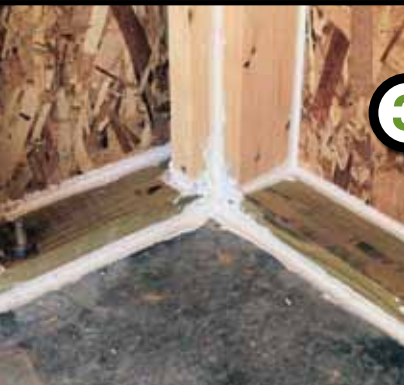
Caulk-sealed bottom plates
