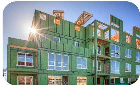
ZIP System® sheathing panels have a single-piece design that makes installation quick and simple. One panel delivers moisture protection and tight air seal, as well as excellent strength and durability. Traditional long length wall sheathing can reduce the number of horizontal joints and the need for
